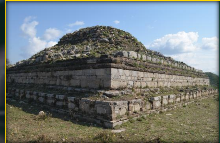
Present view point of Kunala Stupa
